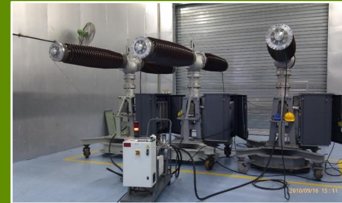
Live tank breaker assembly and testing complying with latest quality and EHS standards
