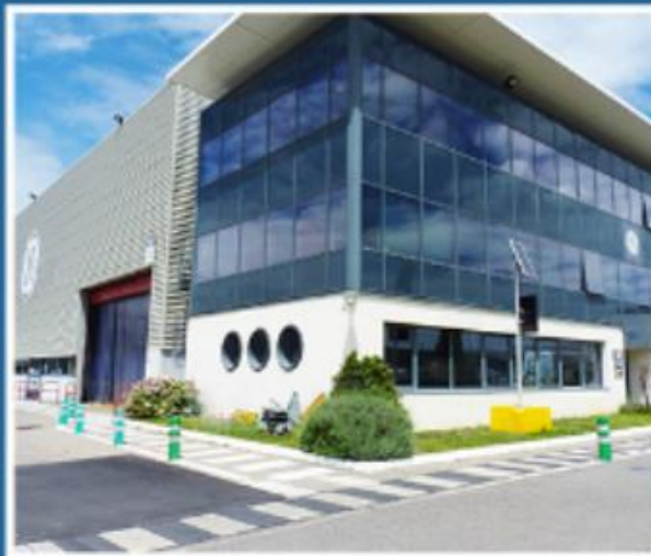
Villeurbanne site includes R&D activities, switchgear manufacturing, test labs and service activities
