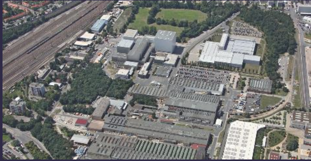
Large Power Transformers Nuremberg Germany
