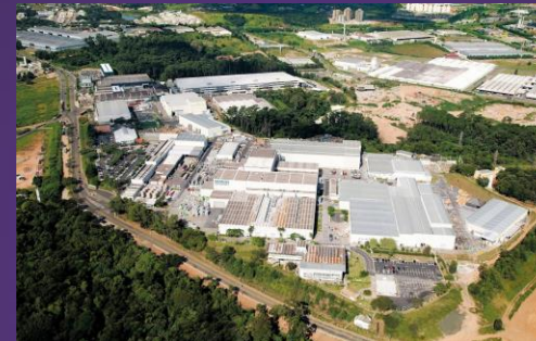
Large Power Transformers Jundiai Brazil
