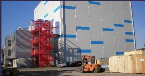
Large Power Transformers Zagreb Croatia
