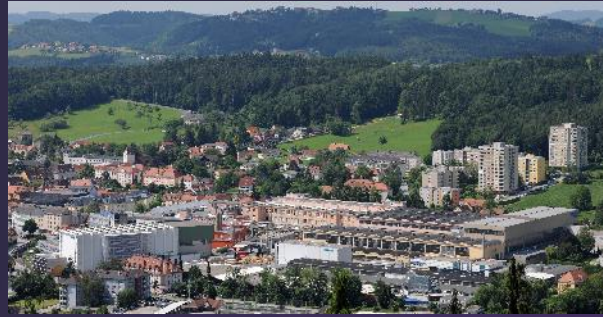
Large Power Transformers Weiz Austria
